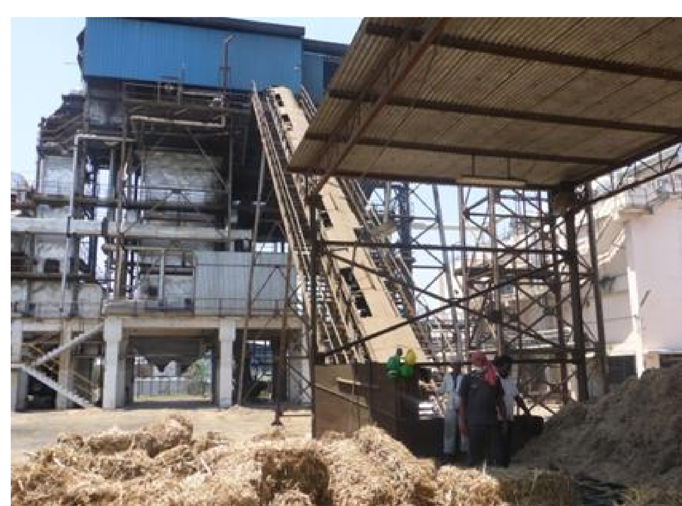
Figure 2. Biomass feeding system of a power plant.
