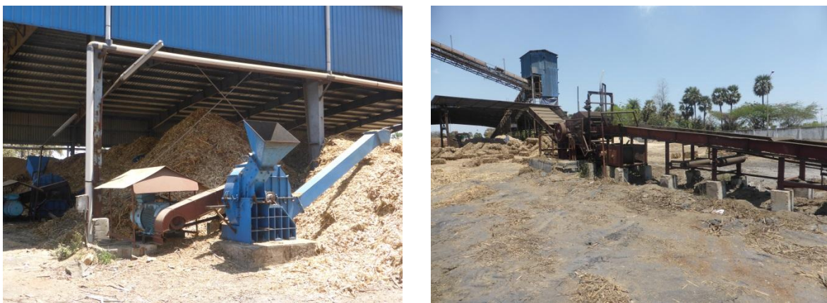
Figure 53. Chipping of Prosopis juliflora (left) and shredding of energy grass and sugar cane trash at power plant (right).
