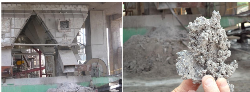
Figure 48. Ash removal system in the boiler (left) and agglomerated ash (right) (Karthikeyan Natarajan).
