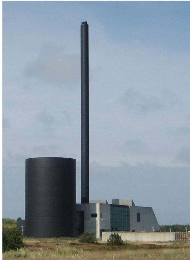
Figure 3. Skagen CHP plant in Denmark. The plant includes a heat accumulator (on the left) and three W28SG engines (Photo: [http://skagensiden.dk/skagensiden/Nybyggeri/\\_Fotoasp/Img\\_2053.jpg](http://skagensiden.dk/skagensiden/Nybyggeri/_Fotoasp/Img_2053.jpg)).
