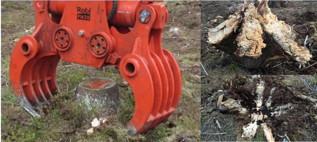
Figure 19. Soil disturbance and impurities can be minimized leaving roots in place.
