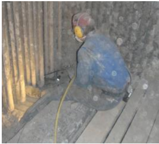
Figure 7.2. Ash removal using compressed air
