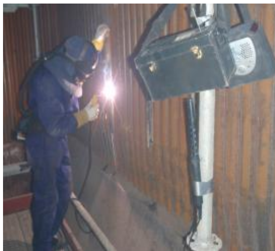
Figure 7.3. Welding of superheater tubes
