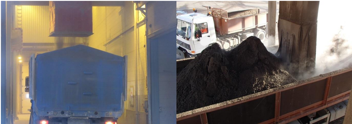
Figure 8. Loading of moistened fly ash to trucks indoors and outdoors.
