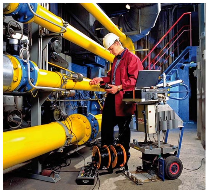
FIGURE 3. Flow meter calibration with tracer technique on a natural gas line.
