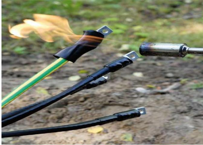
Figure 2.3. LV cable termination using lugs and heat-shrink tubes. (Ensto, 2011)
