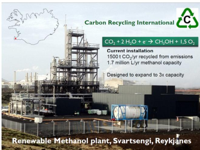
Figure 8 Carbon recycling International's 1.7 million litres per year renewable methanol producing plant (Sigurbjörnsson 2013).
