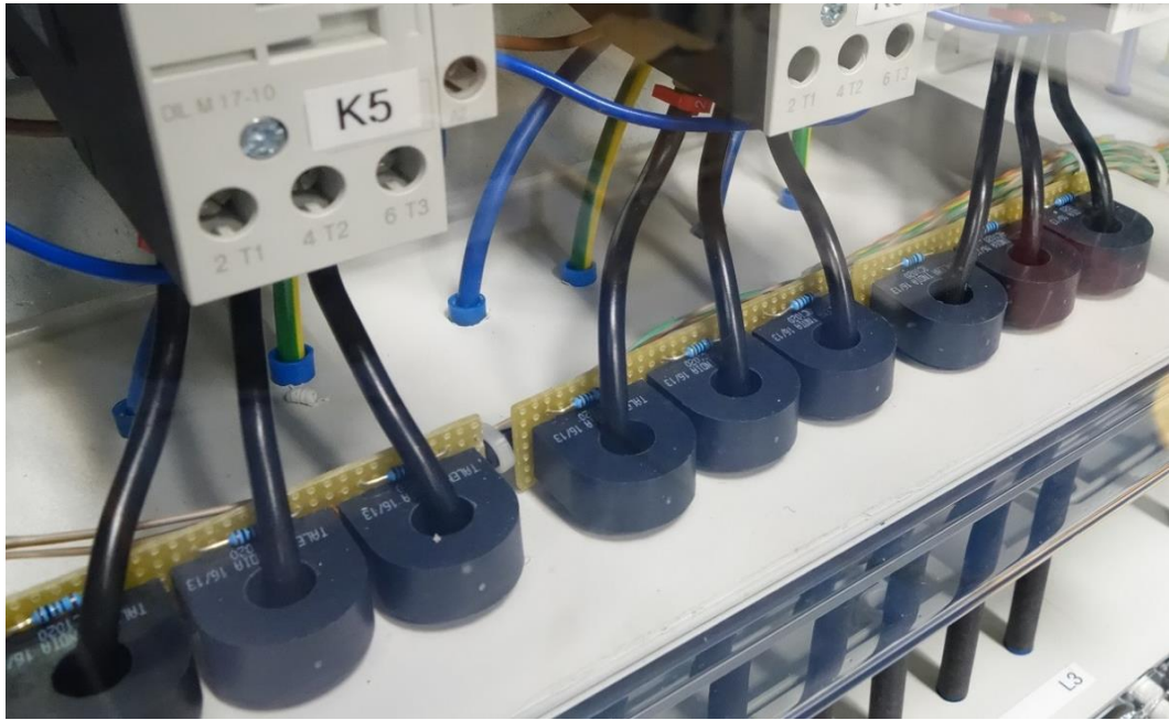
Figure A.3 Photo of three-phase current transducers
