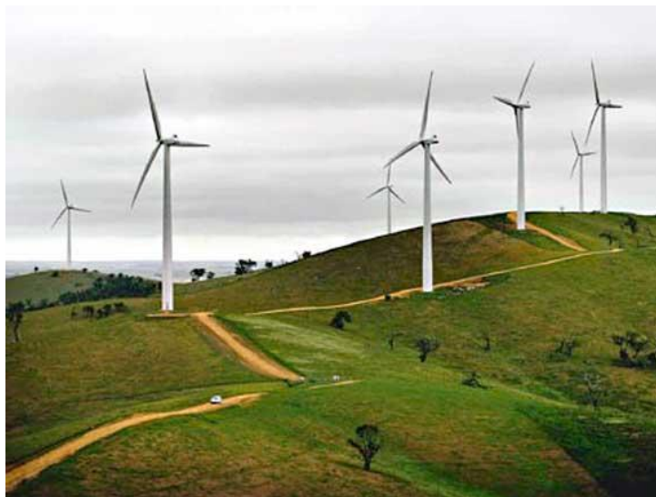
Fig. 1.2. Onshore wind farm in USA [2].
