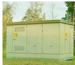
RENOVATION OF DISTRIBUTION TRANSFORMER
