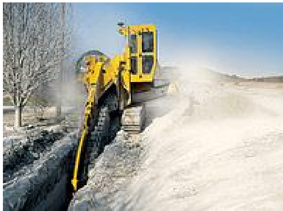
3. Use of chain excavator
