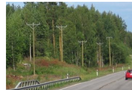
OH-line to roadside
