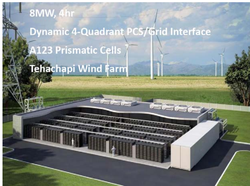
Figure 5-48. An example of the currently started project 8 MW, 4hr li-ion battery system in 660 MW wind power farm in California [Source: A123 Systems].
