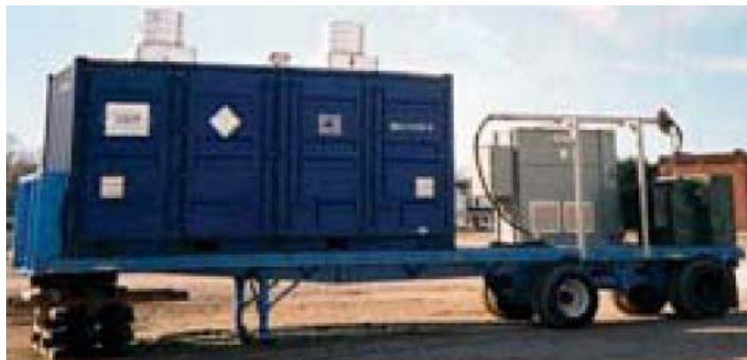
Figure 5-25. 500 kWh transportable Zn-Br storage system [Source: ESA/ZBB].
