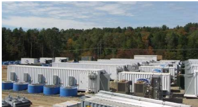
Figure 4-10. 20 MW, 5 MWh flywheel storage plant for regulation services in Stephentown, NY [63].
